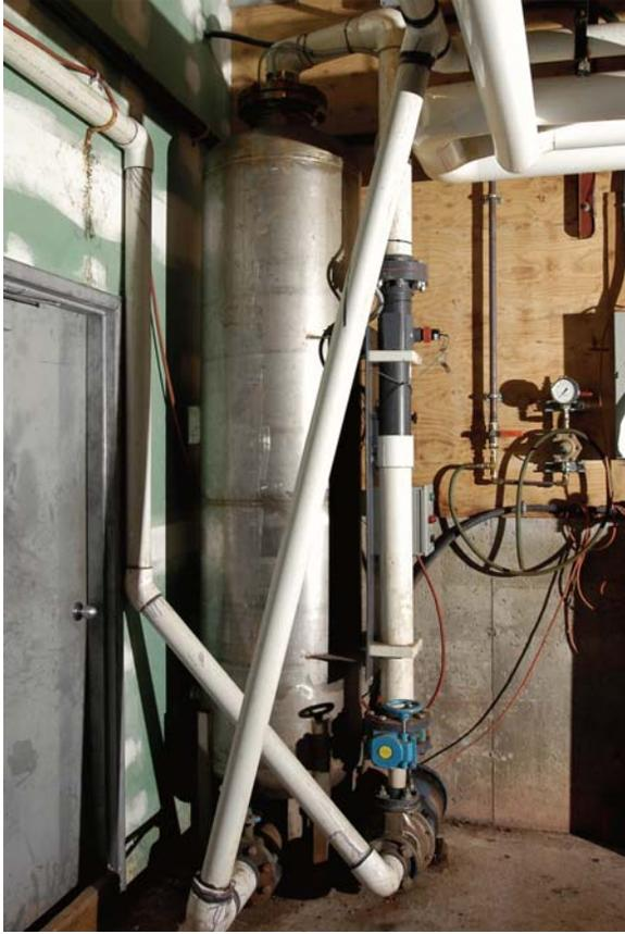
**Figure 6. Pressurized packed column. Note the pump on the floor supplying water to the column.**
