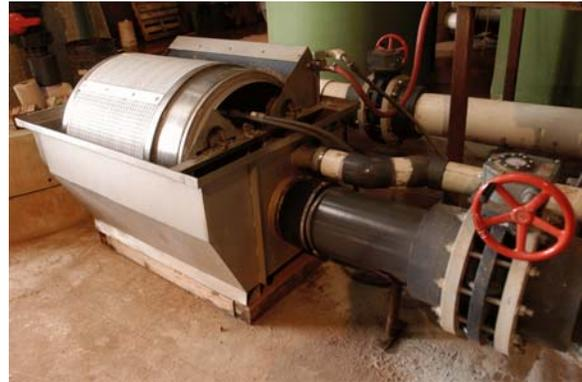
**Figure 4. Rotating microscreen drum.**
