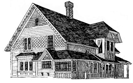
By the 1920s, some houses were being clad in shingles imported from British Columbia. They are much larger, longer-lasting (and thus more expensive) than eastern shingles. Called "Royals", they are sawn from western red cedar and are installed with a 10- to 12-inch exposure.
