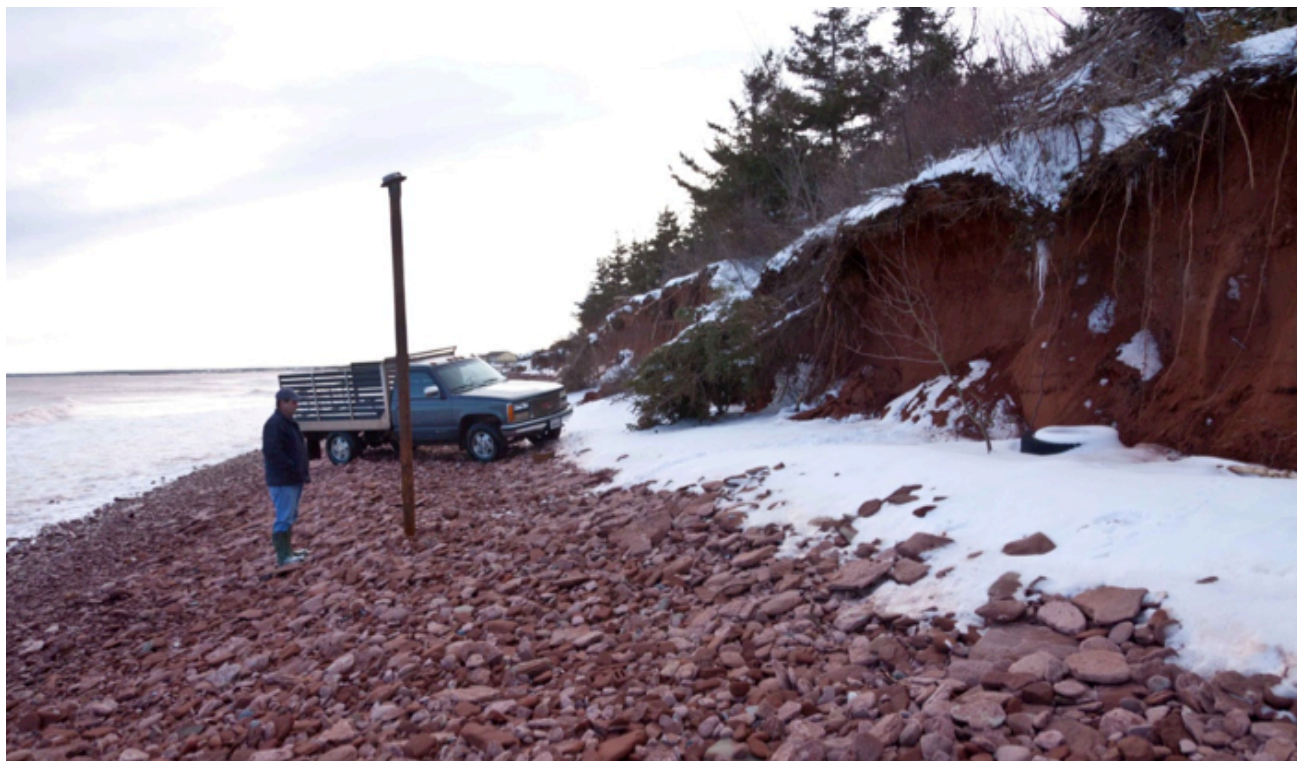
Figure 6. Well relocation. Erosion leaves coastal wells vulnerable to saltwater intrusion as the freshwater-saltwater interface moves inland, occasionally necessitating well relocation. This well, located in Anglo-Tignish, PEI, demonstrates the need for prudence and foresight when drilling wells near the shoreline. (Source: D. Jardine)
