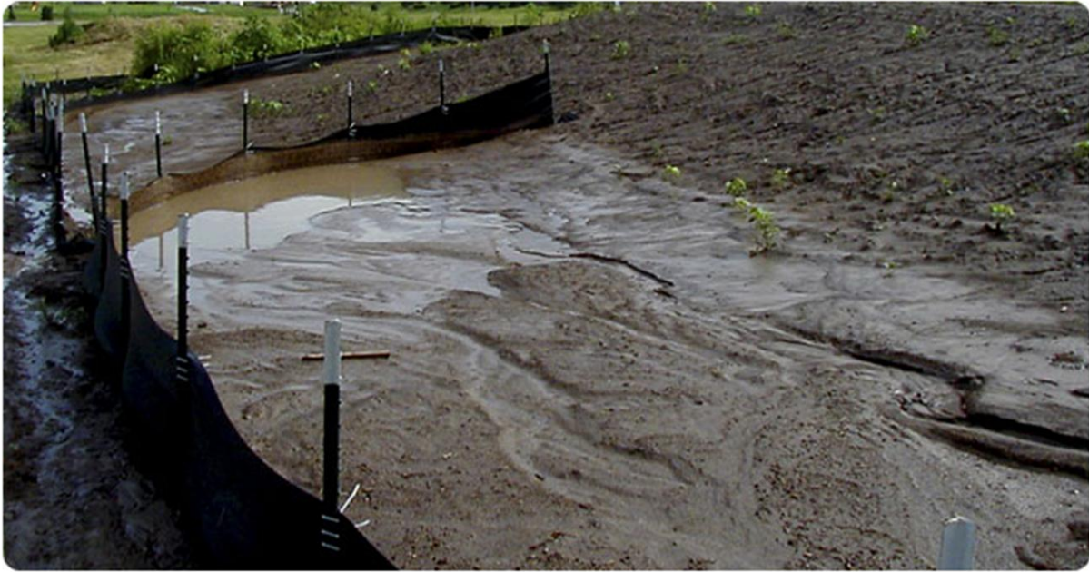
Silt Fence Installed in “J Hook” Configuration
