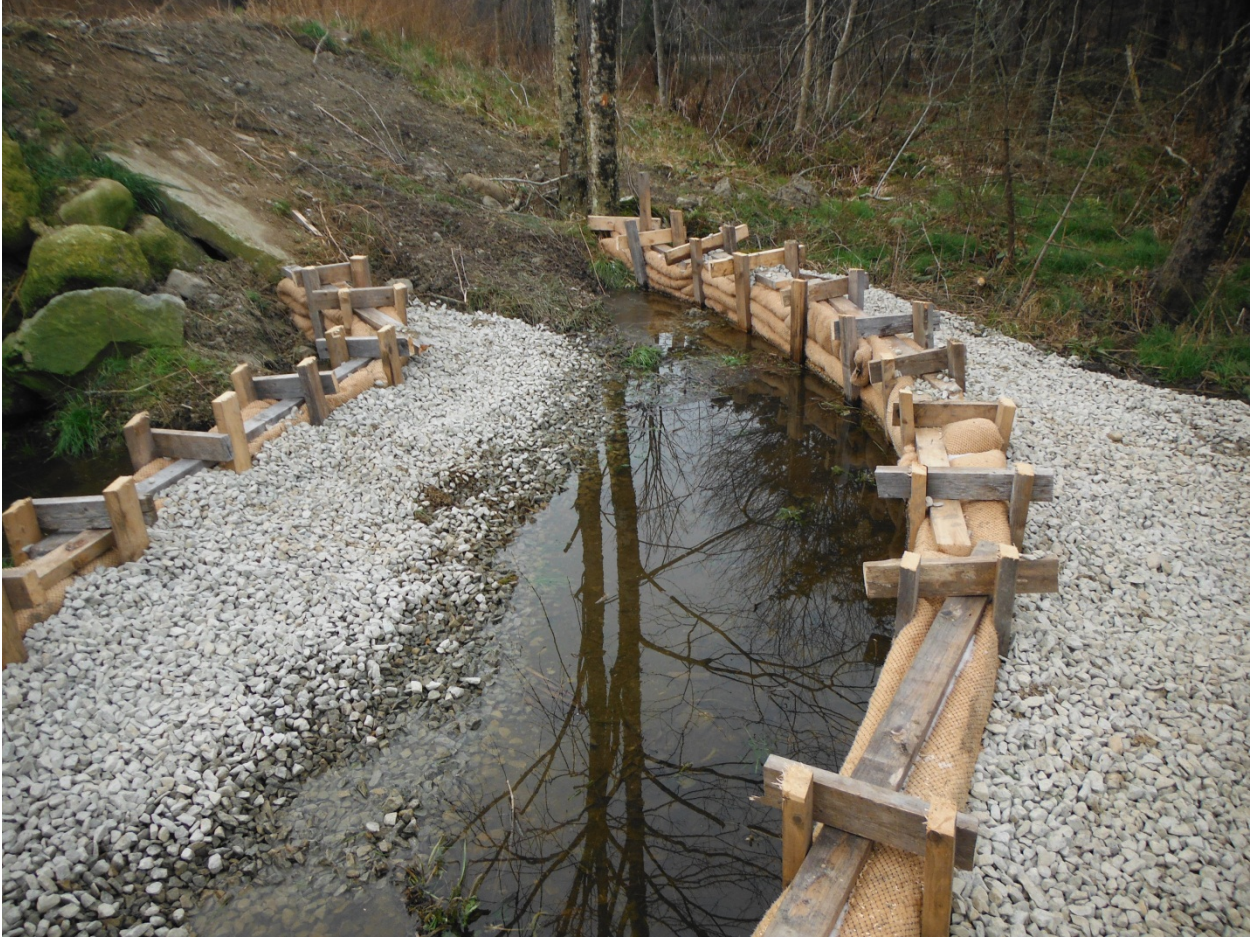
PHOTO 2: Photo showing the final installation of a typical filtration berm.
