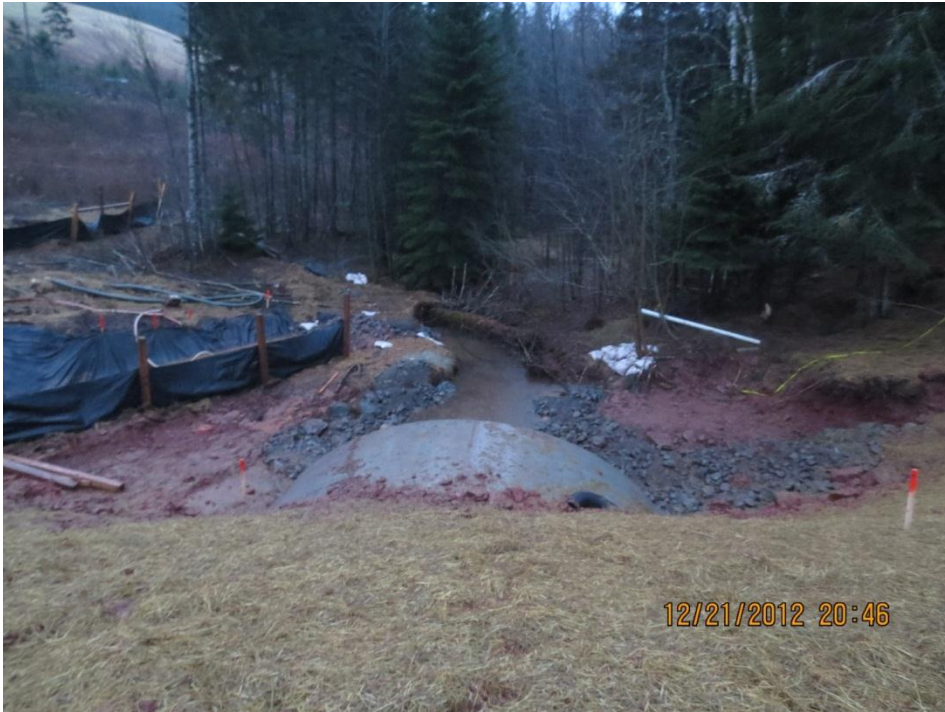
PHOTO 23: Stream flowing through concrete arch at Crawford's Stream (Station 1+500, facing south), December 21, 2012.
