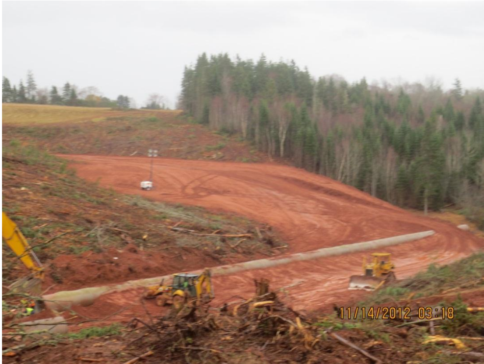
PHOTO 9: Installation of concrete pipe at Encounter Creek (Station 2+400), facing east) November 14, 2012.
