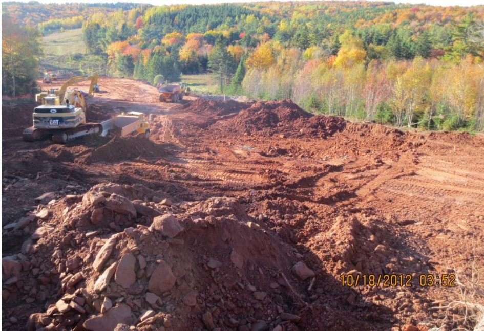
PHOTO 15: Excavation at Crawford's Stream (Station 1+850, facing west), October 18, 2012.
