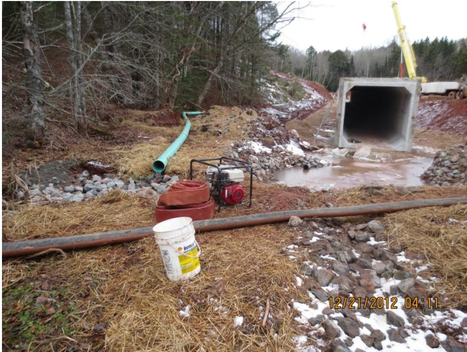
PHOTO 27: Stream diversion pipe and construction of concrete box at Crawford's Brook (Station 1+000, facing north), December 21, 2012.
