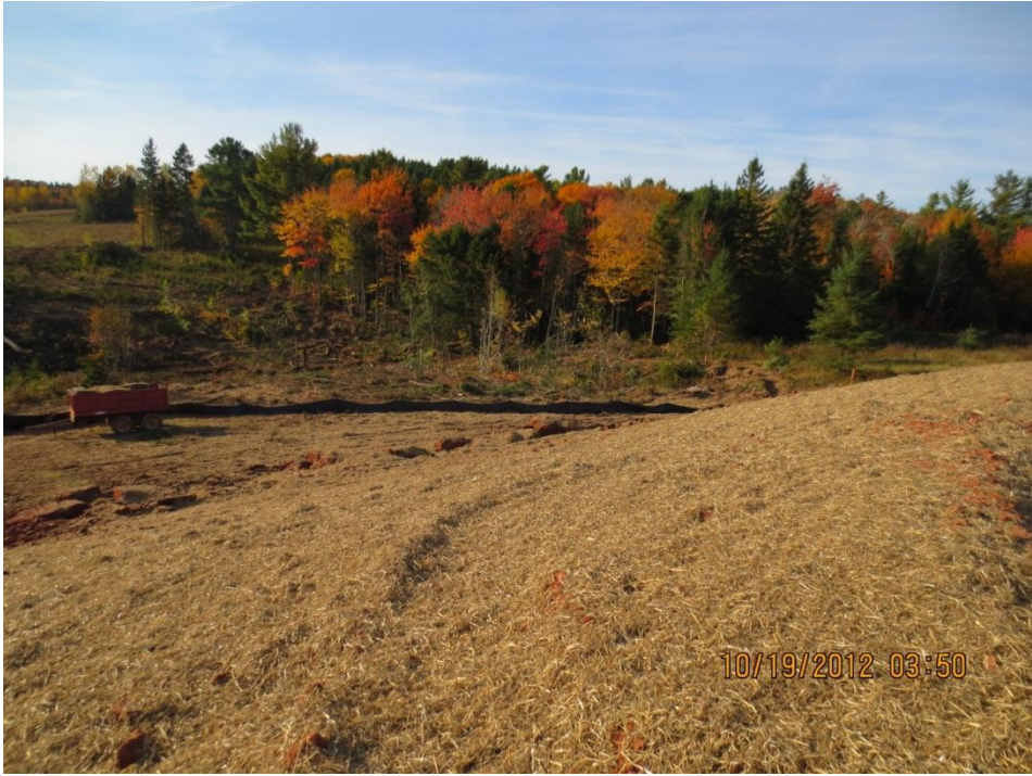
PHOTO 17: Sediment and erosion control at Crawford's Stream (Station 1+550, facing northwest), October 19, 2012.
