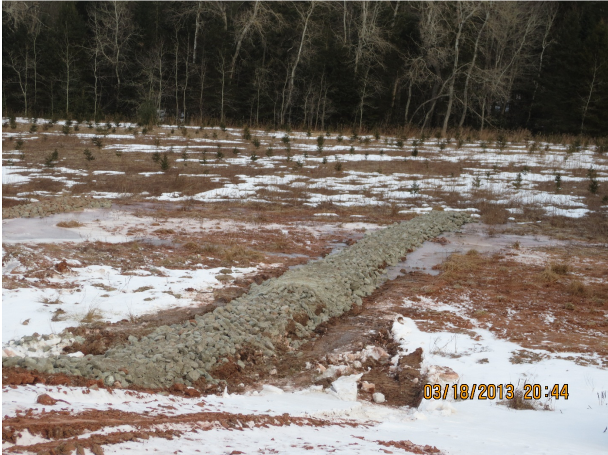
PHOTO 1: Newly constructed rock berm on southeast side of Crawford's Stream, March 18, 2013.
