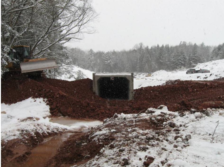
PHOTO 27: Stream diversion pipe and construction of concrete box at Crawford's Brook (Station 1+000, facing north), December 21, 2012.
