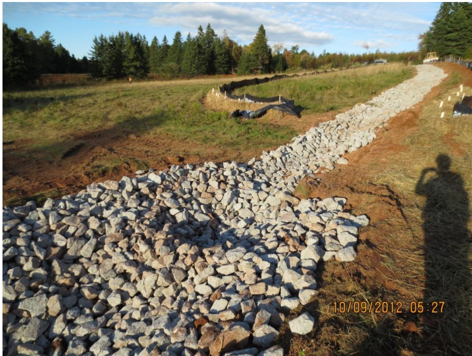
PHOTO 11: Installation of silt fence at Crawford's Stream staging area (Station 1+550, facing west) prior to construction, October 4, 2012.
