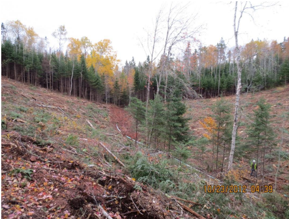
PHOTO 5: Installation of diversion pipe at Encounter Creek (Station 2+450), facing north) October 23, 2012.
