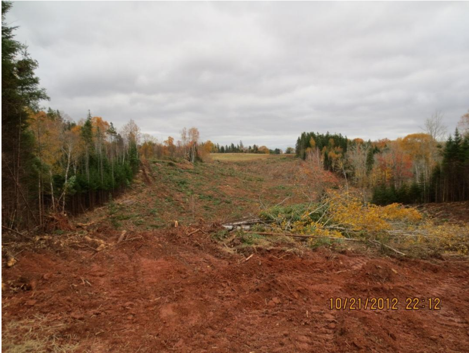
PHOTO 3: Grubbing at Encounter Creek (Station 2+350, facing east), October 21, 2012.
