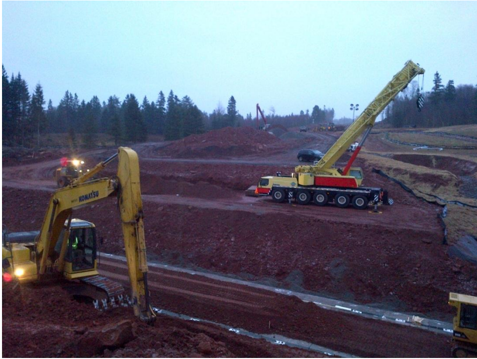
PHOTO 21: Construction of concrete arch at Crawford's Stream (Station 1+450, facing east), December 3, 2012.
