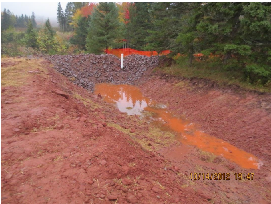
PHOTO 14: Construction of sediment pond at Crawford's Stream (Station 1+550, facing west), October 14, 2012.
