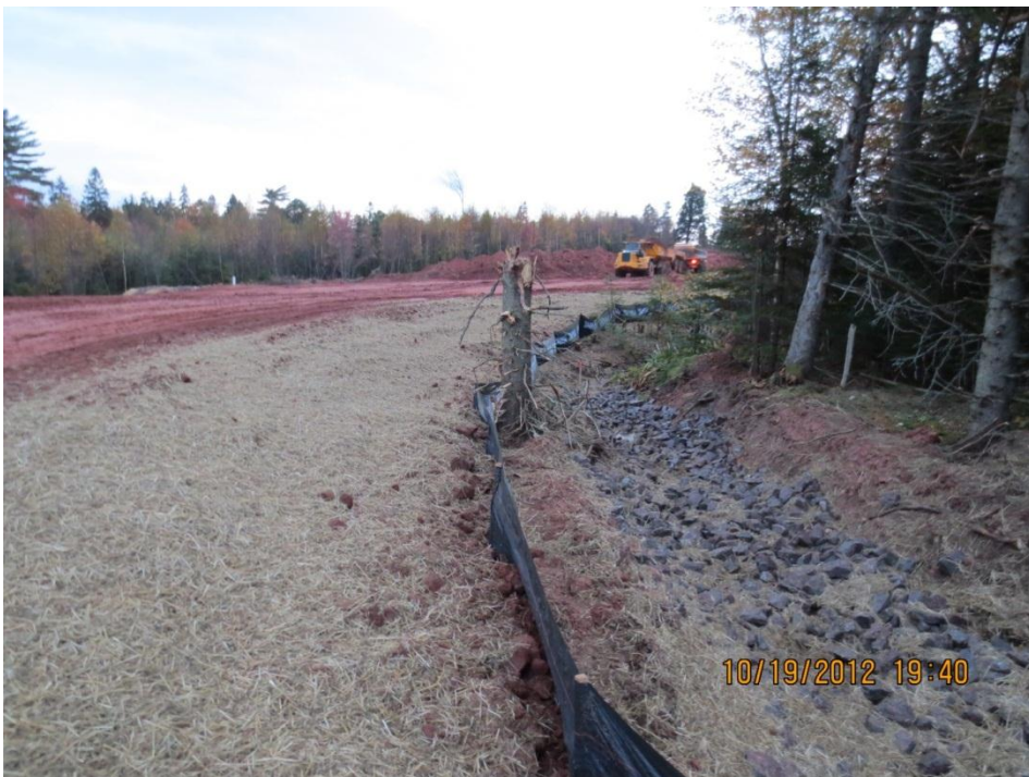
PHOTO 16: Sediment and erosion control at Crawford's Stream (Station 1+640, facing northeast), October 19, 2012.
