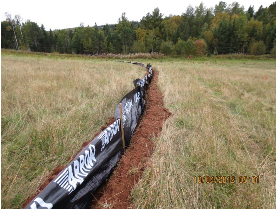
PHOTO 11: Installation of silt fence at Crawford's Stream staging area (Station 1+550, facing west) prior to construction, October 4, 2012.
