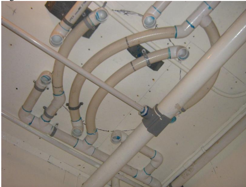
Figure 22: Water inflow distribution manifold seen from below
